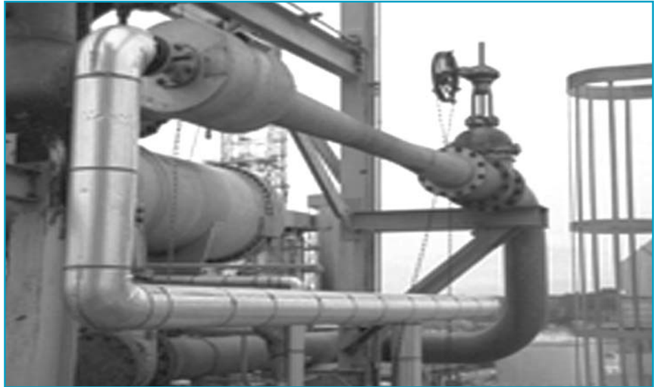
Photo 1 Vacuum Ejector
