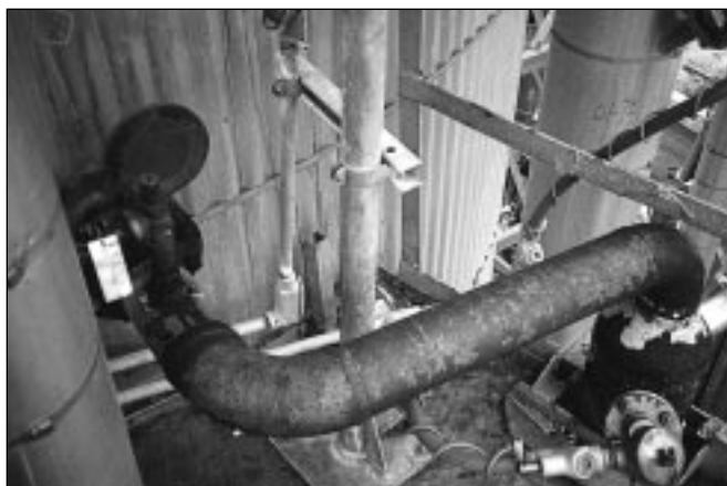
Fig. 9. Pumparound draw nozzle and piping.
