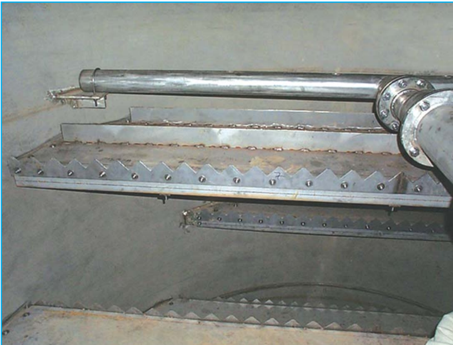
Photo 3. Slurry PA shed trays
