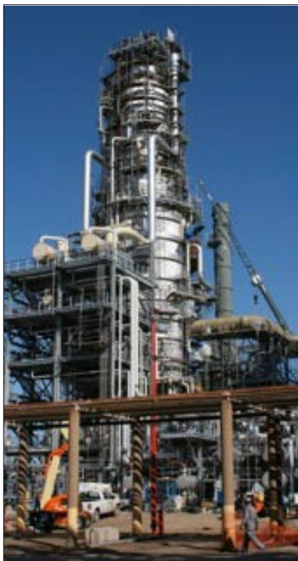
Figure 2 Deep-cut VGO vacuum unit producing diesel from the top draw
