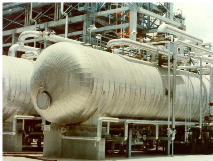
Figure 2 Two Stage Desalter System
