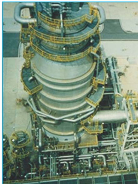
Photo 10. Vacuum Transfer Line
