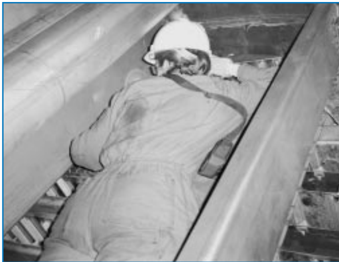
Photo 1 Thorough Packed Column Internals Inspection
