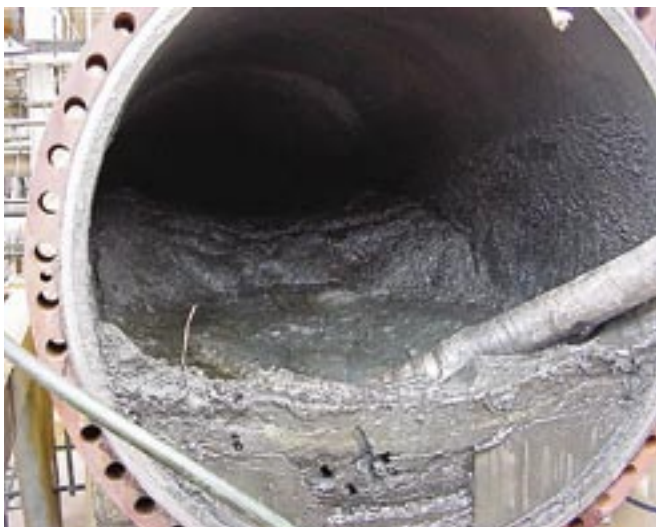
FIG. 13 Salt and corrosion products in top pumparound exchanger shell.
