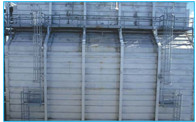
Photo 2. Cabin Heater Side-wall
