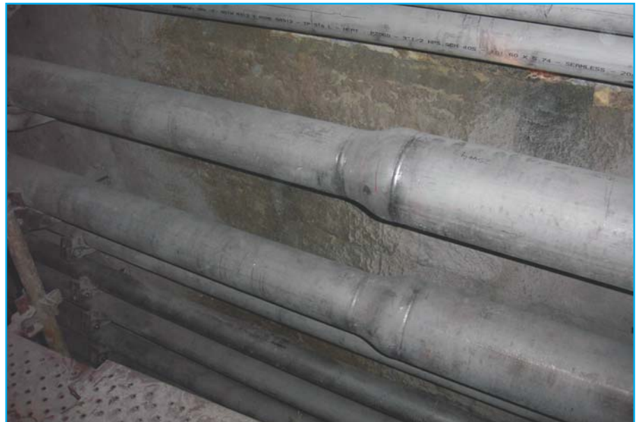
Photo 6. Tube Transition 8" to 10"
